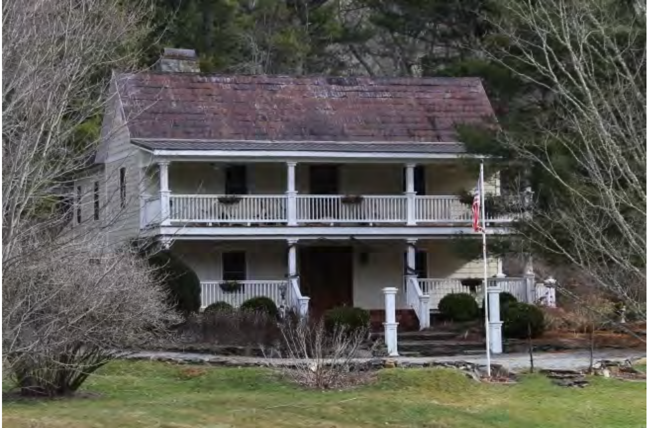
Trivette House (WT 353), 142 Cub Ward Road, façade, view to northeast
