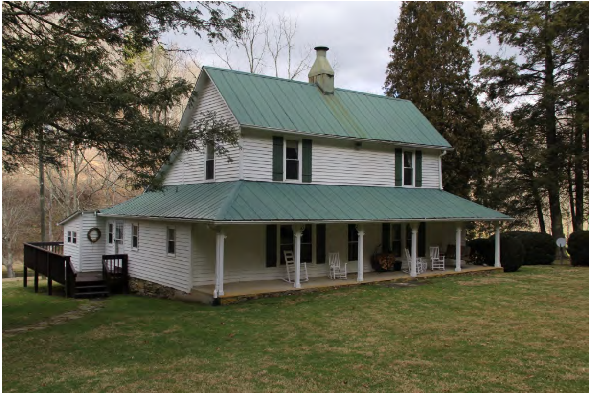
Rubin Walker House, oblique view to north
