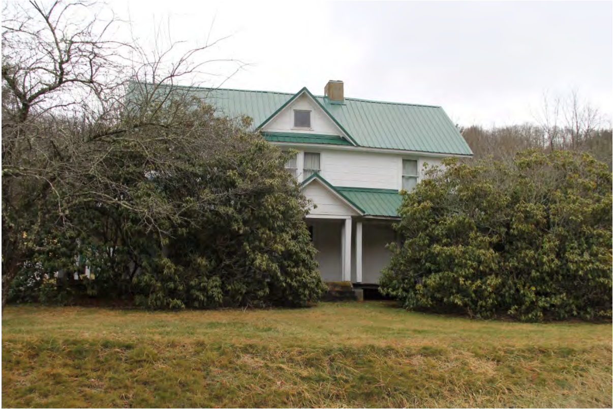
Richardson House (WT 344), 3146 Bairds Creek Road, façade, view to east
