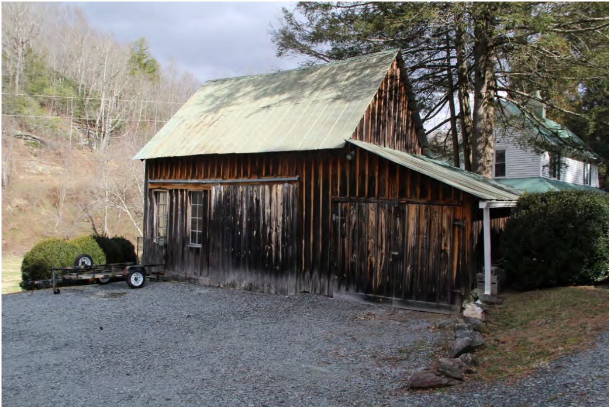
Barn, southeast elevation, view to northwest
